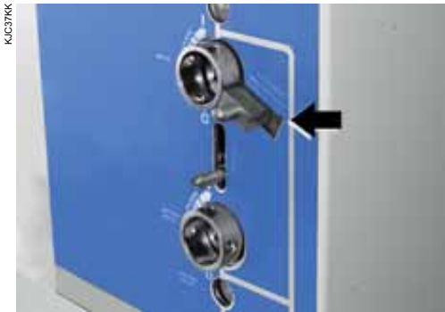
Disconnecter control operation interlock device
